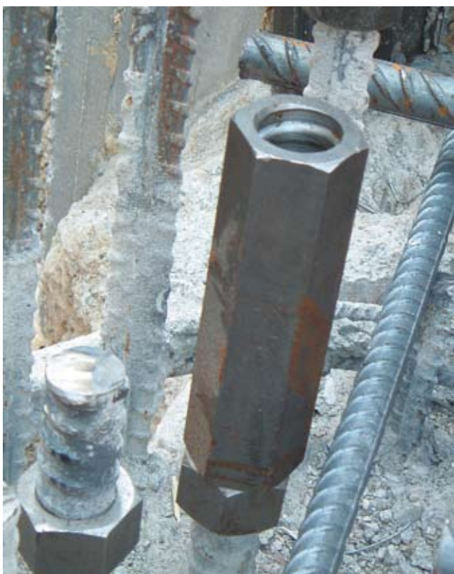
Muffenverbindung (Stab-Ø 32 mm) coupler connection (bar-Ø 32 mm)
